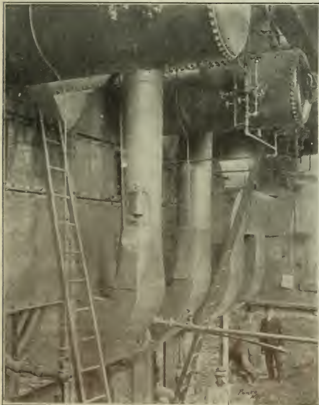
BOILER FRONTS DURING CHANGE
